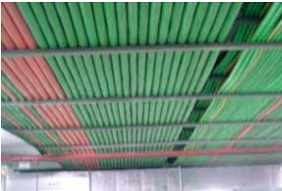
Installation of EXZHELLENT XXI and SEGURFOC-331 SECTORFLEX® type, 4x120 mm 2 composite cables.
