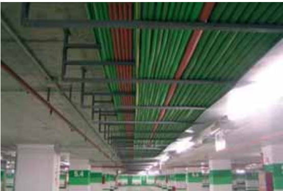
Installation of EXZHELLENT XXI and SEGURFOC-331 SECTORFLEX® type, 4x120 mm 2 composite cables.
