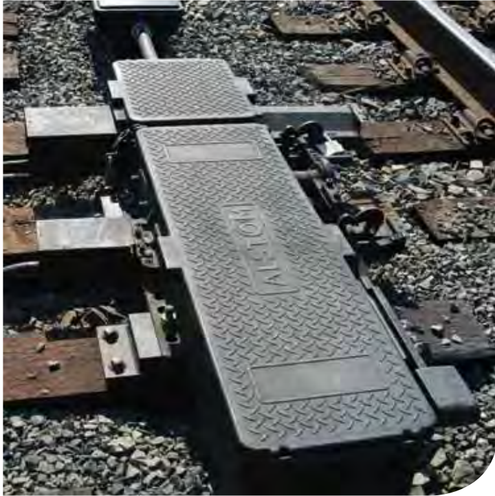
GM4000A™ Switch Machine installed at customer location
