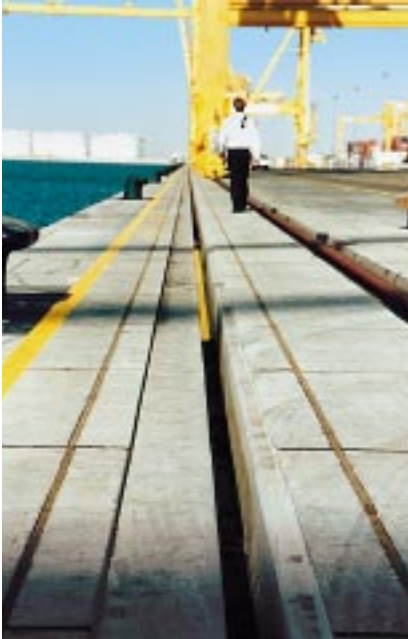
Jebel Ali Port - Dubai. The pre-existing slot used for the Panzerbelt® installation.
