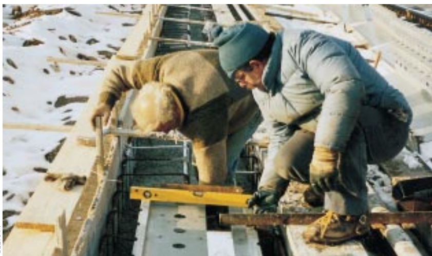
7 Positioning of belt and fixing through the pre-drilled steel strip using rivets.
