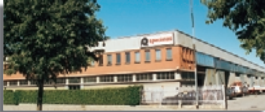
The Specimas plant in Italy
