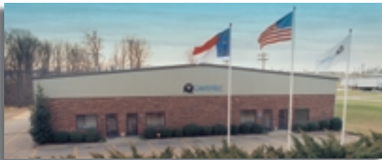
Offices and plant of the Cavotec company in the USA
