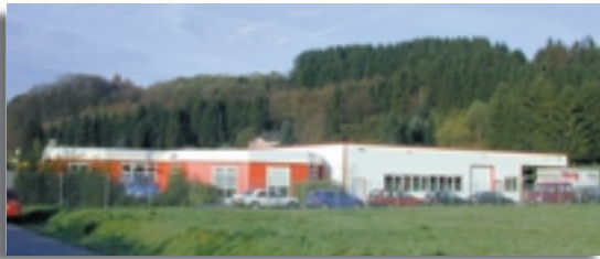
The Alfo Cavotec plant in Germany
