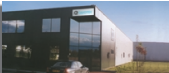
Cavotec RMS in France
