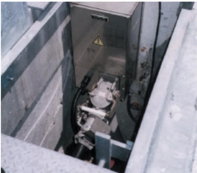
Cranes are often connected to the power line with Cavotec Connectors. The photo shows a Push & Pull Power Socket, including fiber optic socket and connection box.
