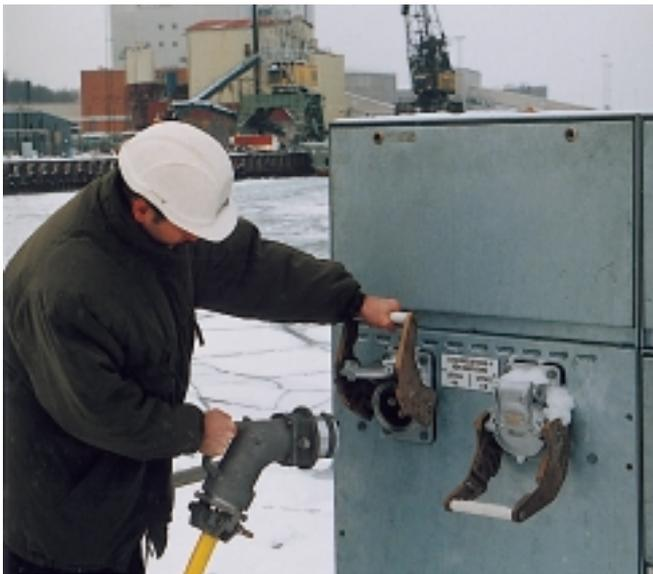
Above two X5-type connectors in the harbour of Stockholm. The unique Push & Pull design assists the operators to connect the plug and socket without effort, also in severe environmental conditions caused by ice, snow, dust, extreme temperatures or corrosive atmosphere.
