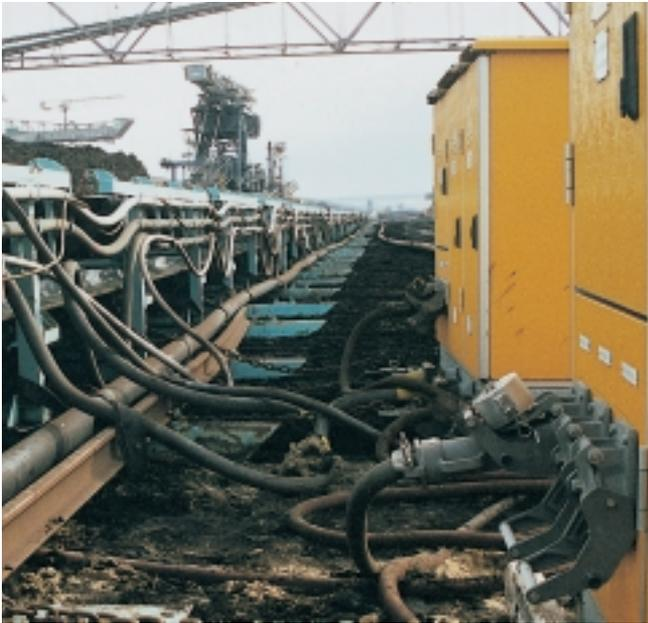
Thanks to their robust design these connectors are often used in harsh environments such as this open pit mine in Germany.
