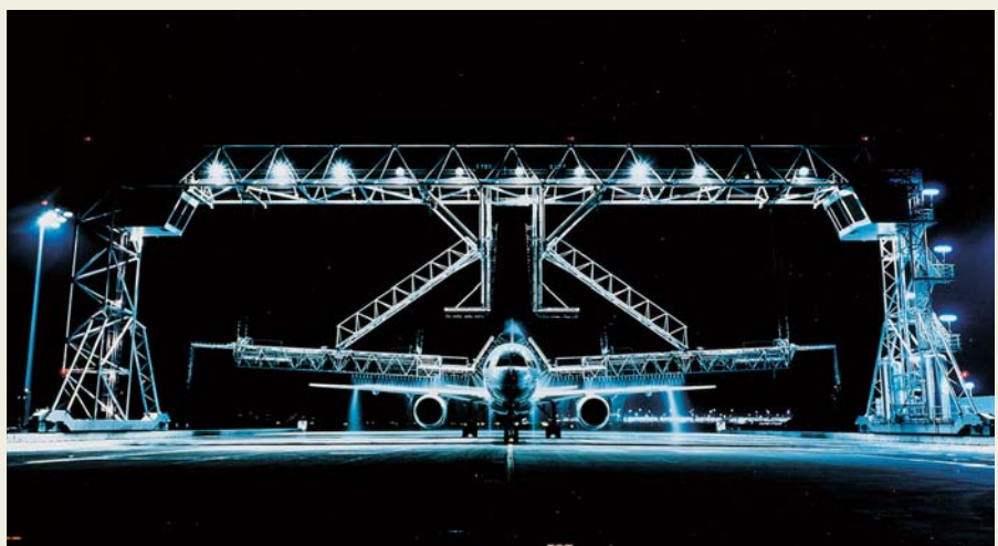
A steel chain application in action on a de-icing installation at Munich Airport.
