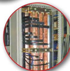
Vertical busbar next to compartments up to 1700 A.
