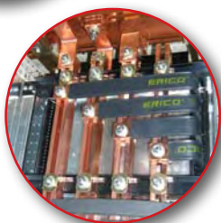
Vertical busbar behind compartments up to 1900 A.
