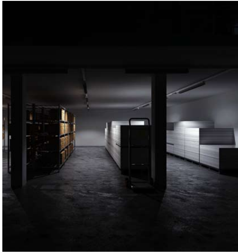
Industrial premises with LED-based emergency lighting.
