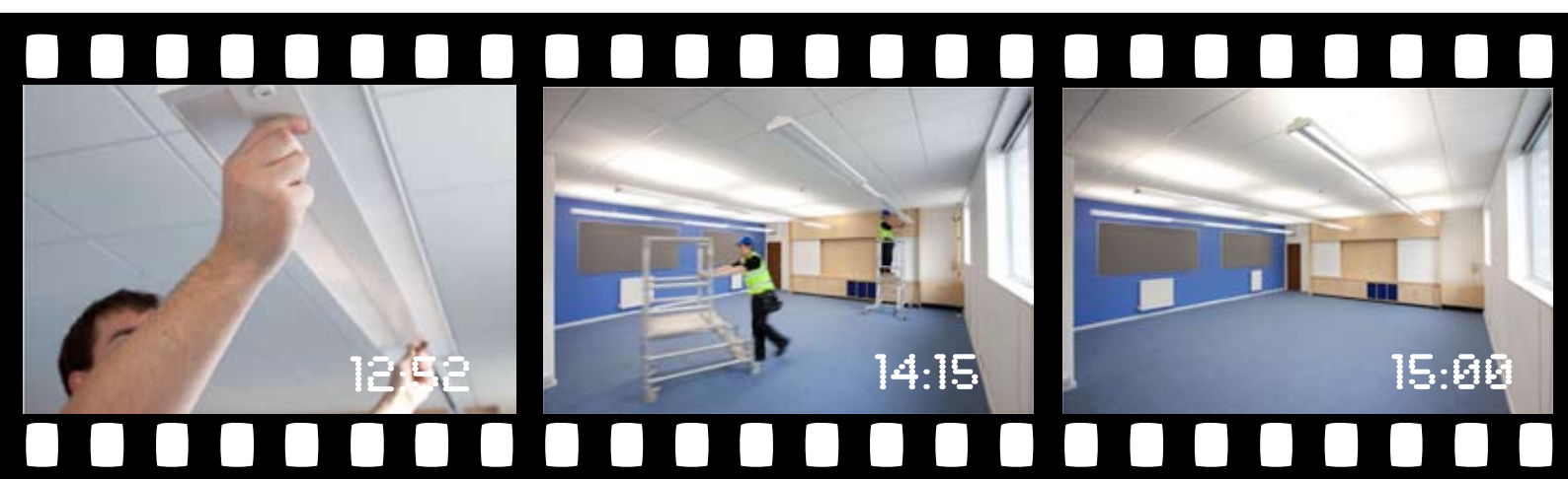
12:52 The luminaires are affixed to the track by means of quick lock.
