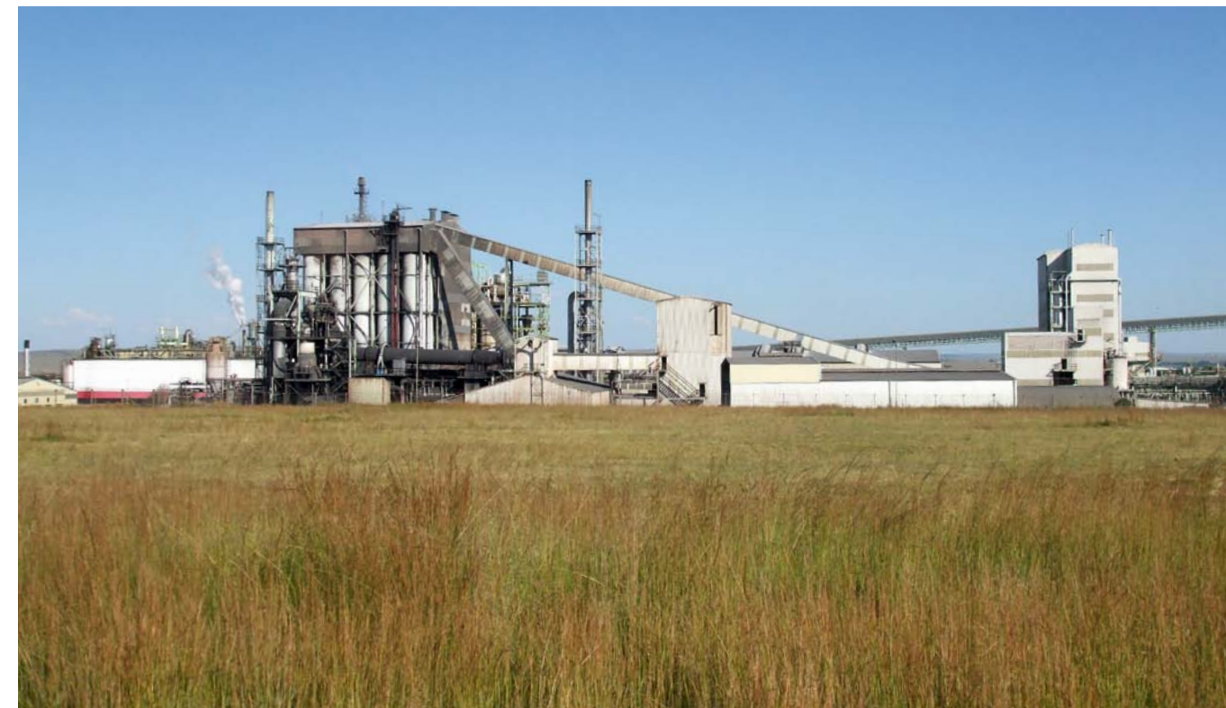
-> THE PRODUCTION FACILITY OF SOUTH AFRICAN CALCIUM CARBIDE (SACC) IN NEWCASTLE, SOUTH AFRICA
