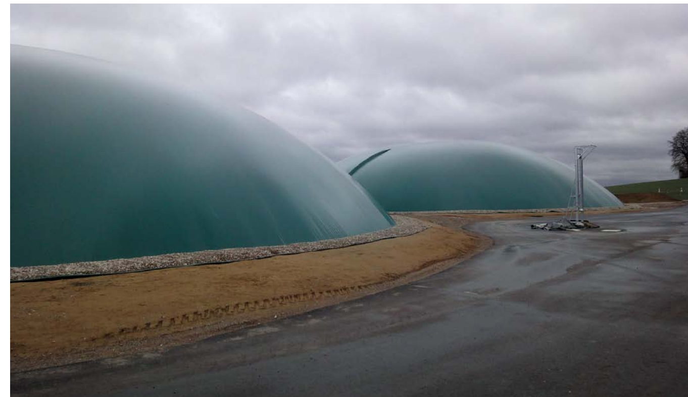
→ VIEW OF THE BIOGAS PLANT IN JEDESHEIM NEAR ILLERTISSEN, GERMANY
