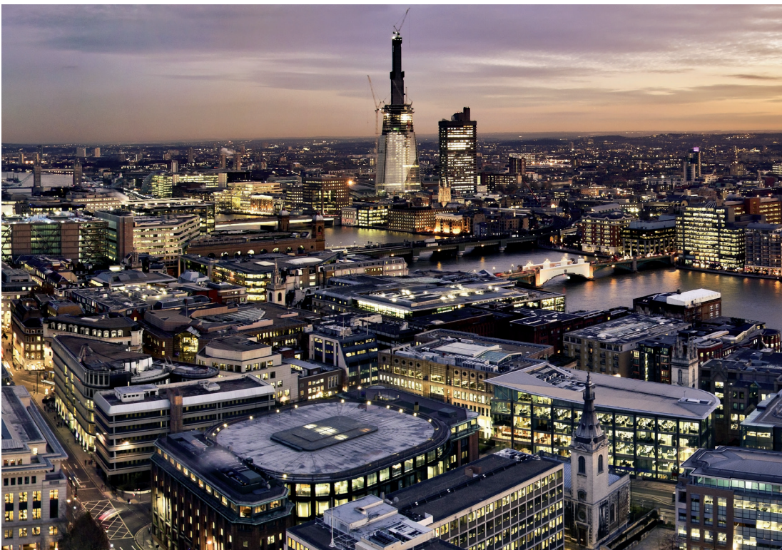
Prysmian Group used 350 km of high-tech fire-resistant cables to enhance the safety of The Shard, Western Europe's tallest building.
