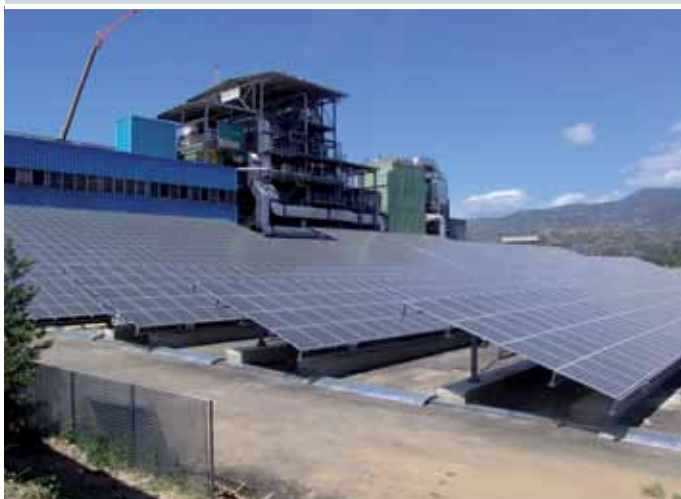
Rende (CS) Potenza impianto: 1,0 MWp EPC Contractor: Siemens S.p.A. - Energy Sector
