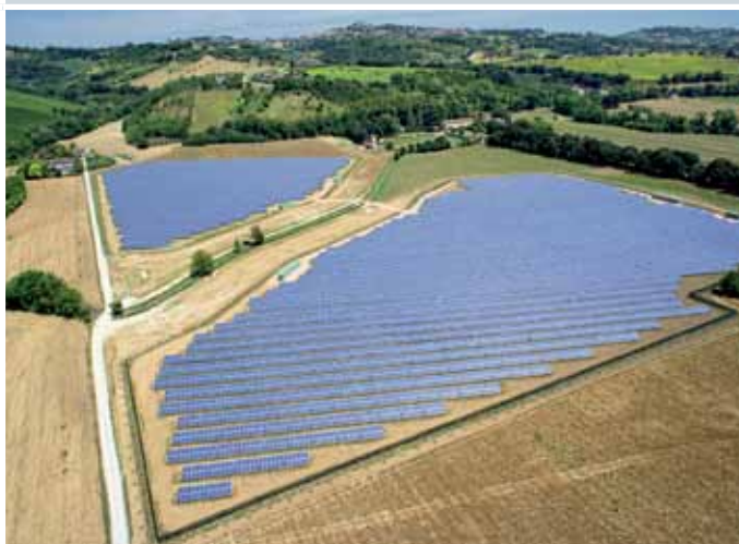
Fontebella (FM) EPC Contractor: Siemens S.p.A. - Energy Sector
