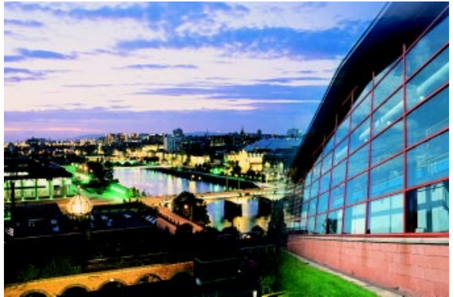
Terasaki Europe Facility
