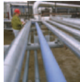
... to preventive maintenance
