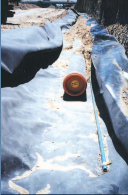
Jet fuel transfer line with blue PVC slotted conduit for TT5000 installed at a major international airport.
