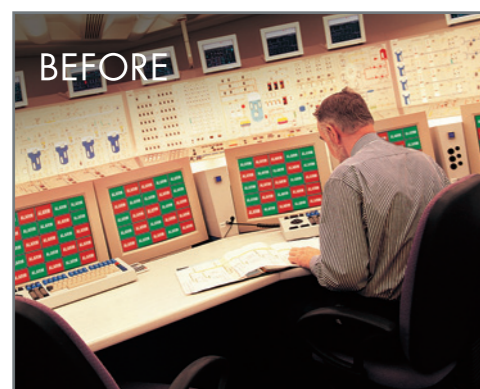
Operators inundated with spurious alarms
