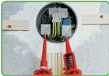
Testing voltage at PUSH WIRE® connectors.
