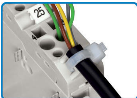
Securing the cable on the connector
