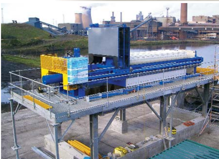
Complete refurbished filter. Addition of booth washer and support structure.
