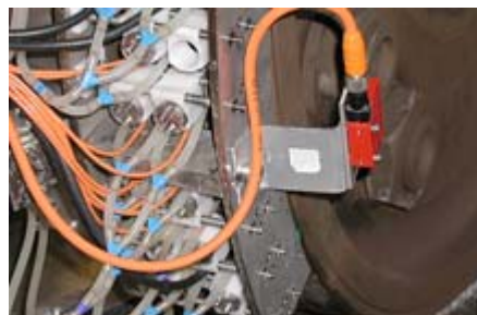
Orientation position inspection
