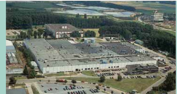
TIENEN (Belgium) for low and standard voltage halogen lamps, discharge lamps and LED lamps
