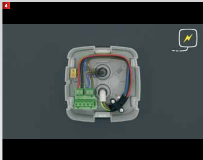
4 Add Vidaflex sleeving, clamp power-in cable and wire-in to terminal blocks.
