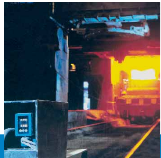
DME measuring the distance of a rail car in a steel mill.
