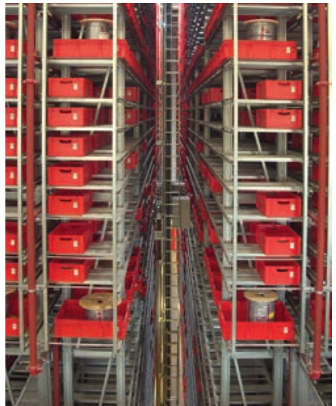
Small parts warehouse
