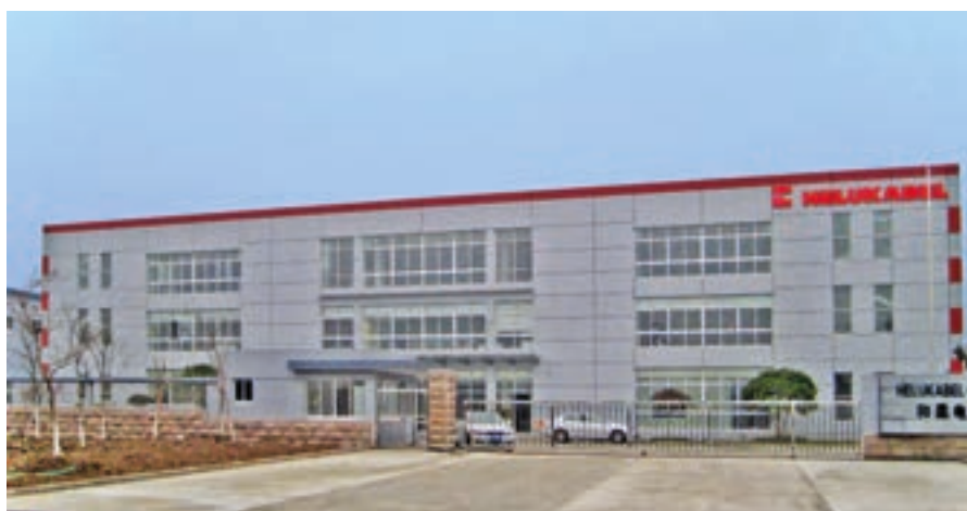
HELUKABEL® Production and Logistics Center in Taicang / China
