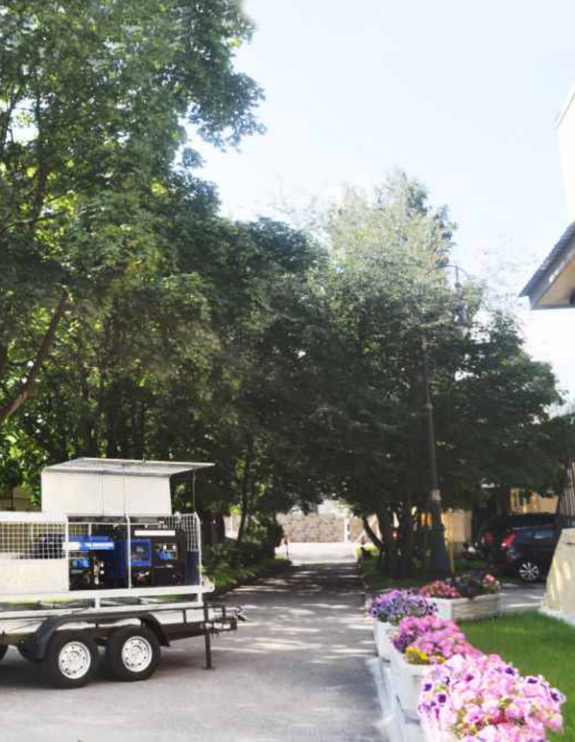
Mobile lighting unit with placement on trailer
