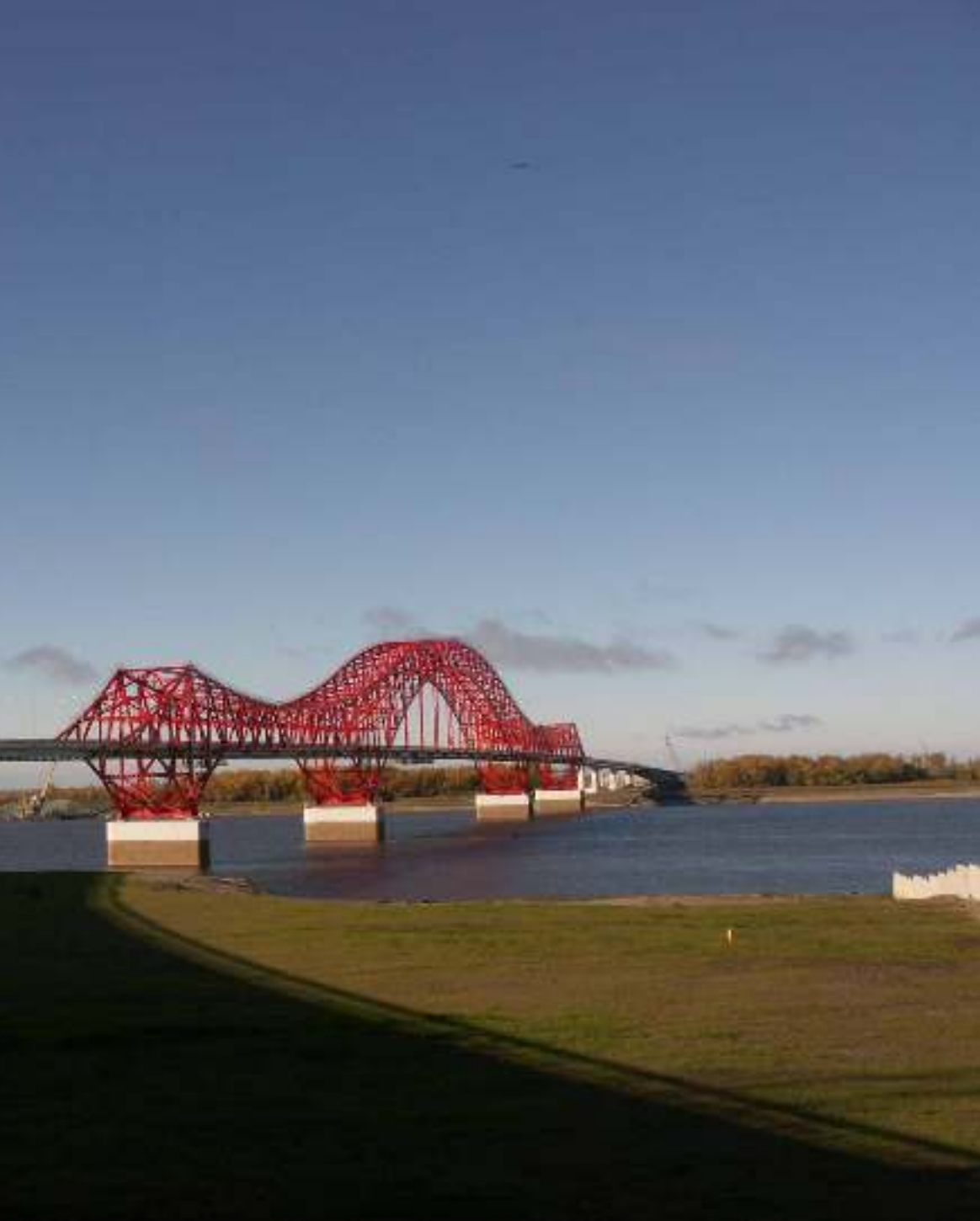
The Bridge across the Irtysh river Ural, Russia
