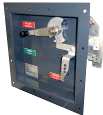
C - Disconnect Inverters
