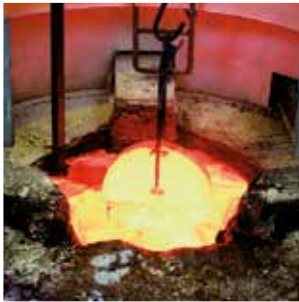
Industrial furnace construction
