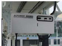
Airport Apron / Hangar
