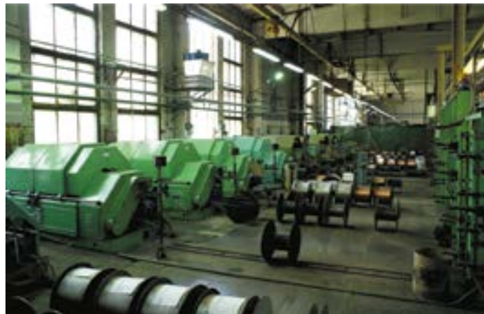
REPAIR- MECHANICAL SHOP
