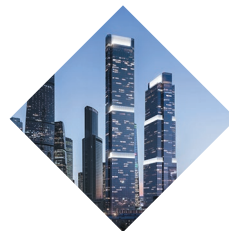
МФК Neva Towers
